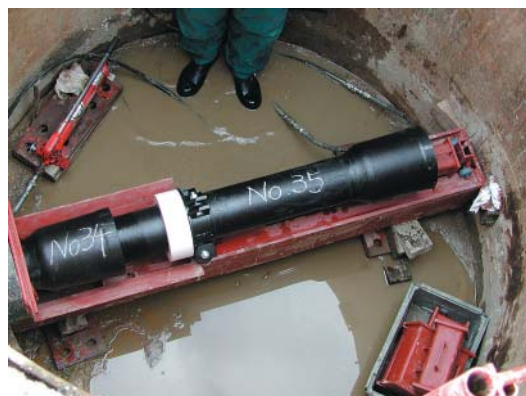
図11 施工状況 Fig. 11 State of construction
