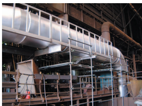
図6 熱風ダクト更新工事 Fig. 6 Renewal construction of the duct for hot blast
