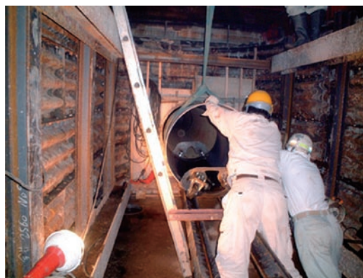
図5 鋼管挿入 Fig.5 Insertion of a steel pipe
