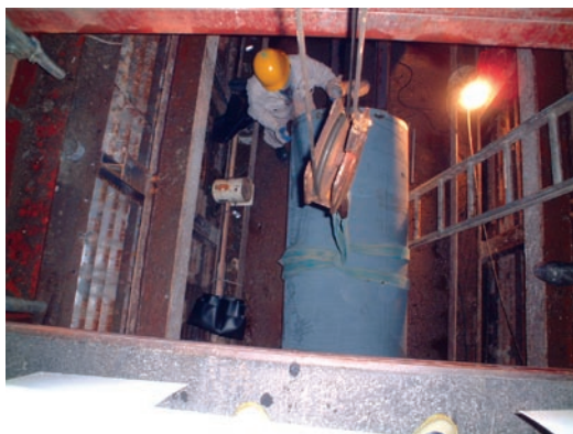
図7 鋼管吊込み Fig.7 Hang a single part of steel pipe
