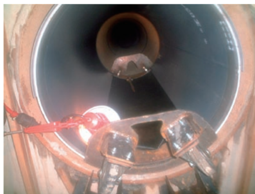
図4 台車取付け状況 Fig.4 Appearance of steel pipe in carriage
